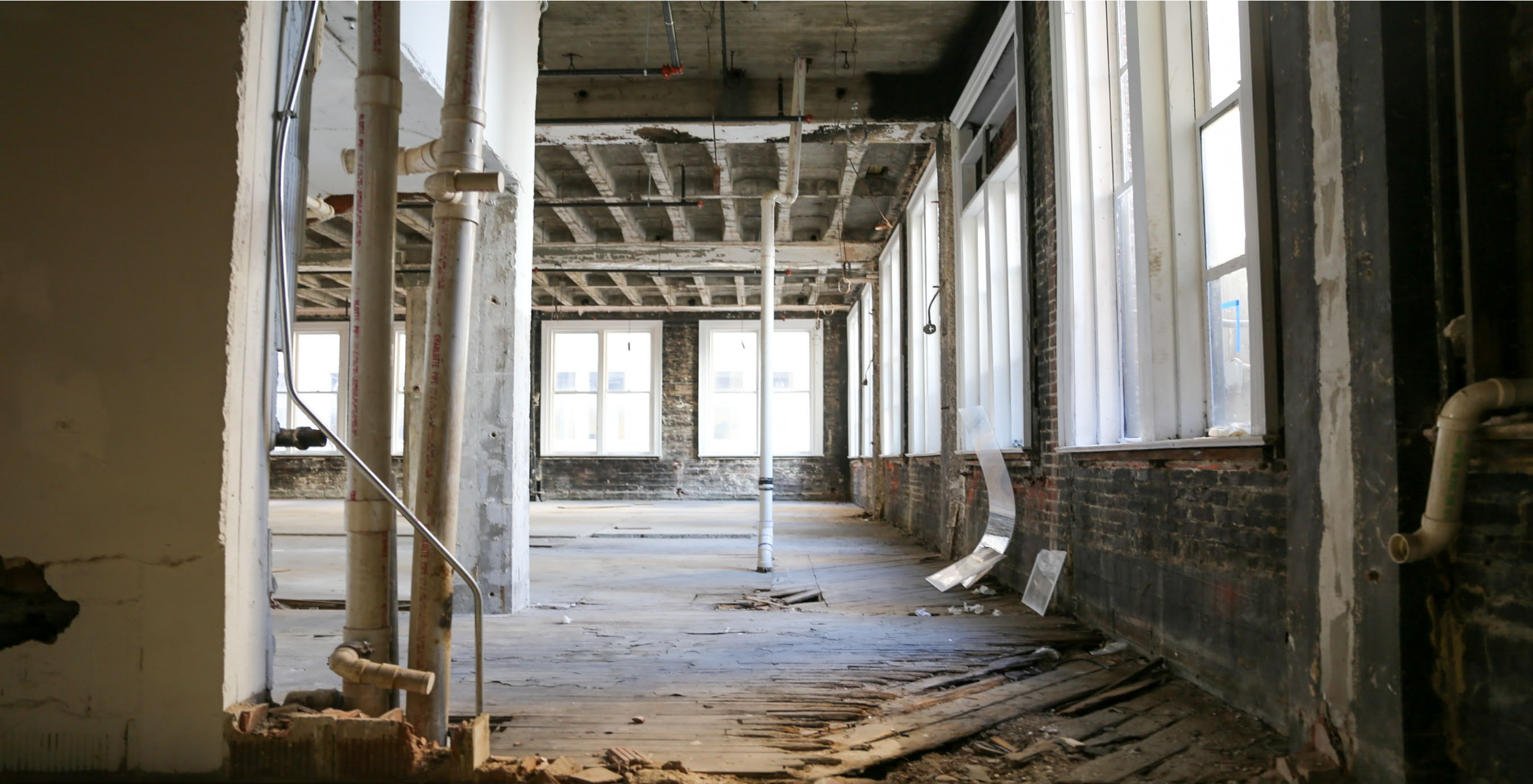
17 ANDREW YOUNG BLVD - 2nd Floor Unfinished Floors
